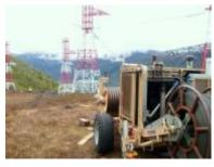
Line construction - SAUDI ARABIA Yanbu-Madinah 380 kV line Longest project portion: 230 km 4-500mm<sup>2</sup> AAAC conductors per phase
