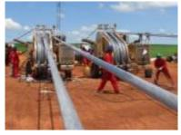
In altitude - PERU 500 kV line at 1000 mt a.s.l., 900 km long 2 modular machines for stringing 4 bundled conductors per phase
