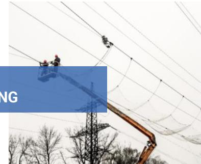
The best solution for installation of safety nets on critical crossings.
