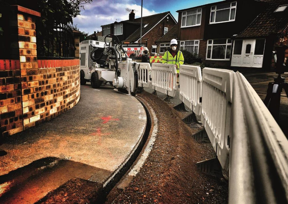
Fiber Optics Laying UK Georadar Explorer 2.0 & Sidecut
