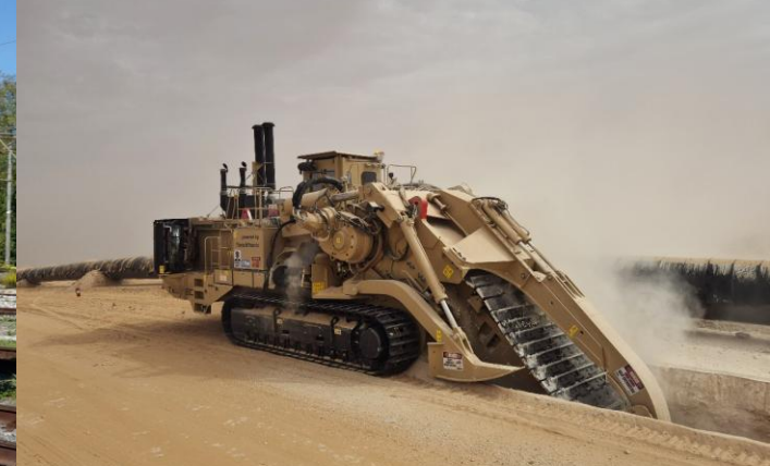
TRENCHER 1875XL EVO GAS PIPELINE
